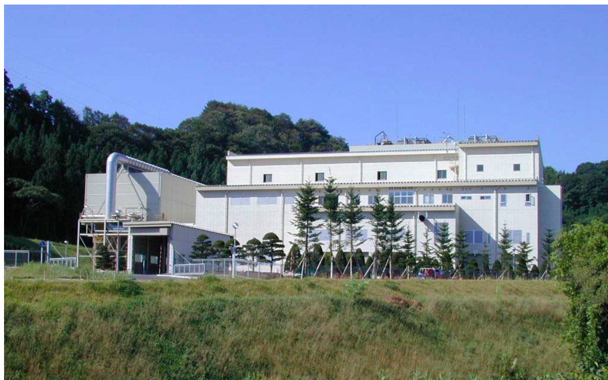
Figure 82. TwinRec facility in Aomori, Japan
