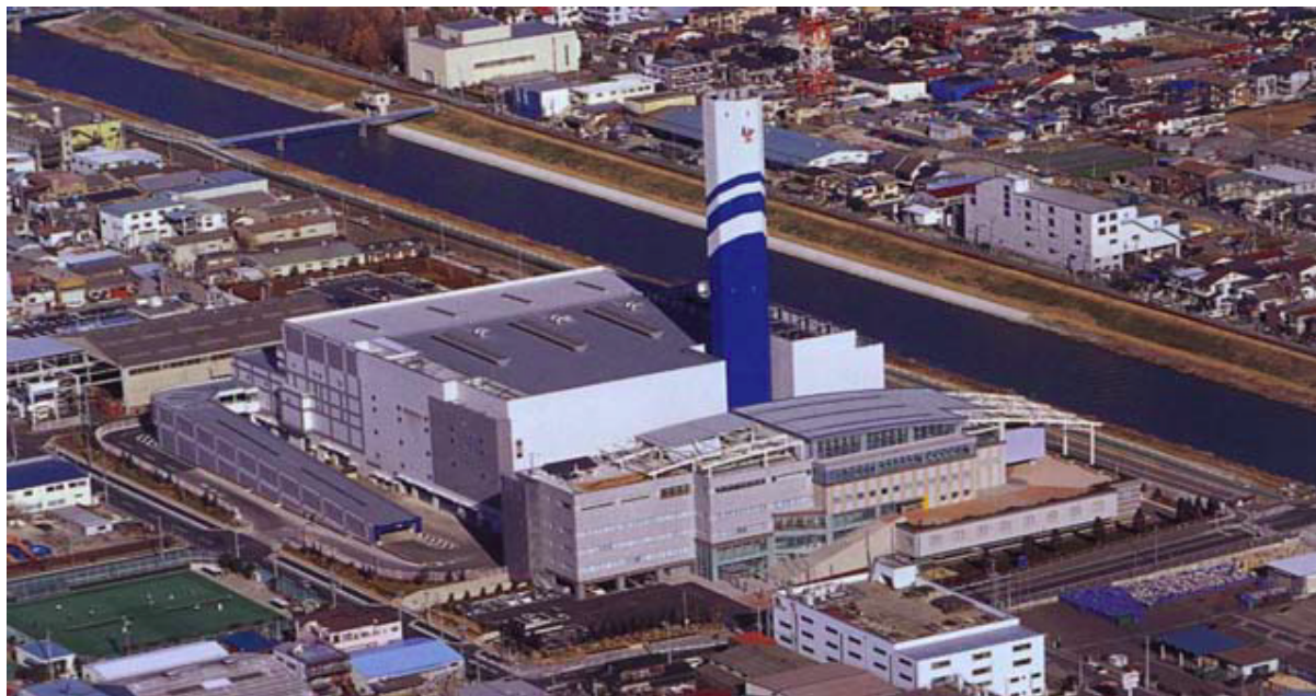
Figure 83. TwinRec facility in Kawaguchi, Japan
